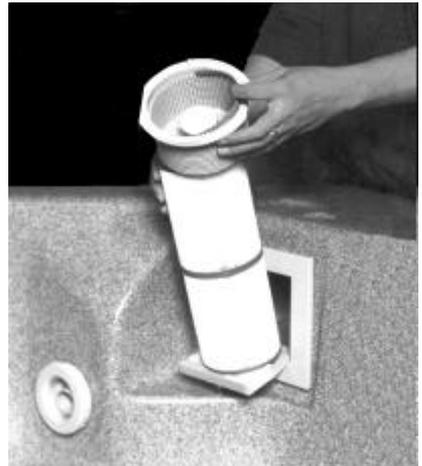
Every 2 months, more often with heavy use, filter must be cleaned to get rid of objects and particles that are lodged in the filter pleats. Using a garden hose with a pressurized nozzle push water from the inside to the outside of the filter pleats forcing all trapped particles out. If the filter is far too dirty to be cleaned as described above, obtain from your dealer filter cleaner material. Soak the filter overnight, then hose it down. Filters will last many years if properly maintained.
